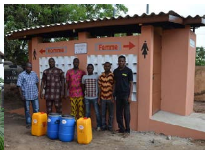
Collection of public waste, co-composting site and public EcoSan latrines
